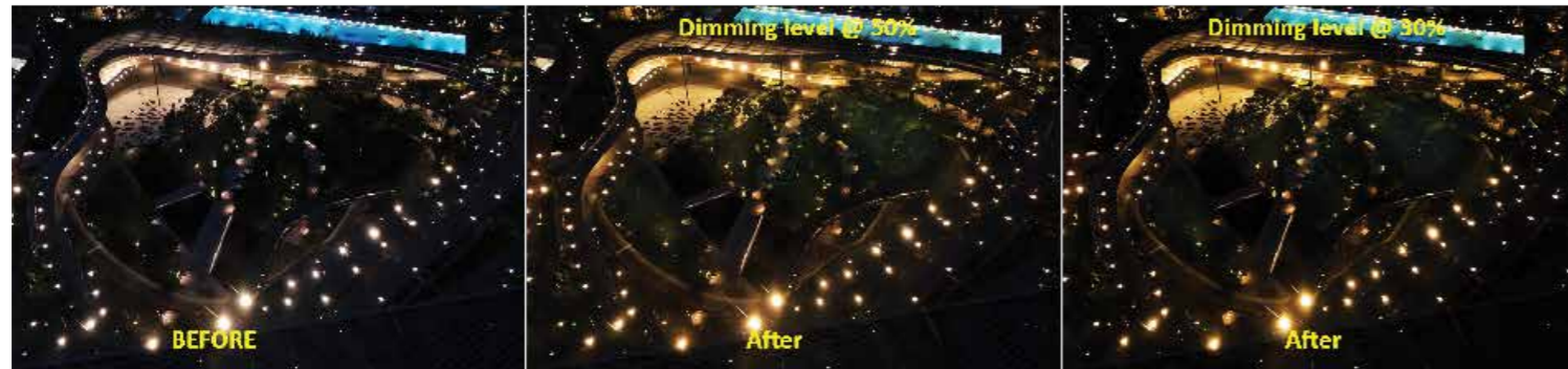
Visualizing illumination levels before installation at the Marina One project.
